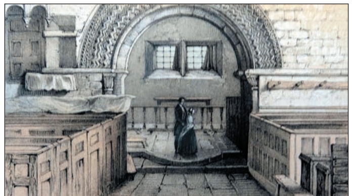
The interior of Yaverland Church as Kilvert will have seen it.
